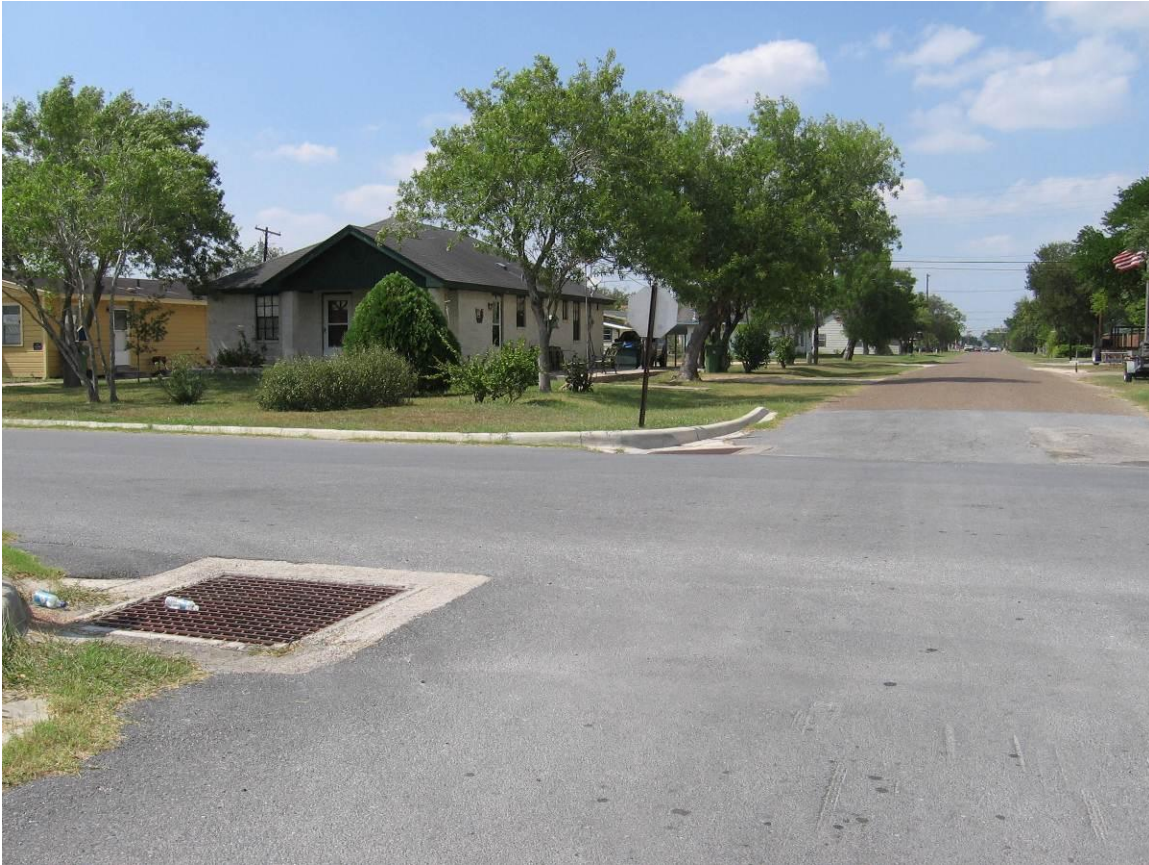
Figure 7D. Area Inlet in good condition
