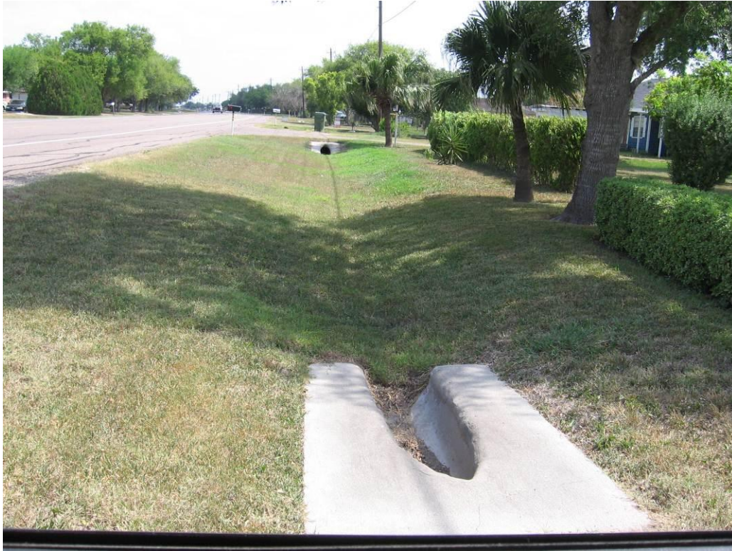
Figure 7A. Roadside ditch along thoroughfare in good condition
