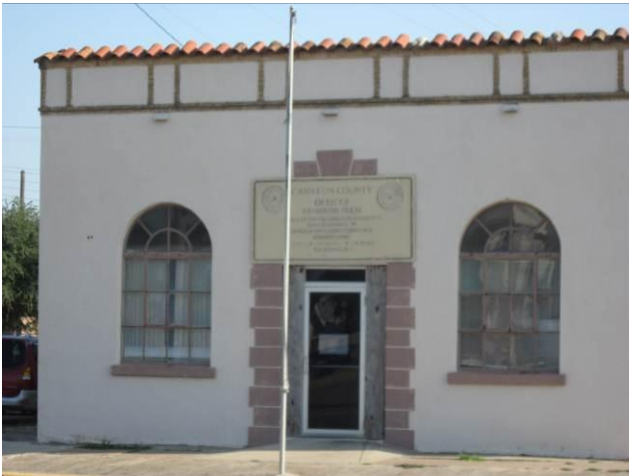
This school and county building constructed in 1994 was sold and remodeled in 2011 as shown (right), changing window shapes, paint colors and glass type.
