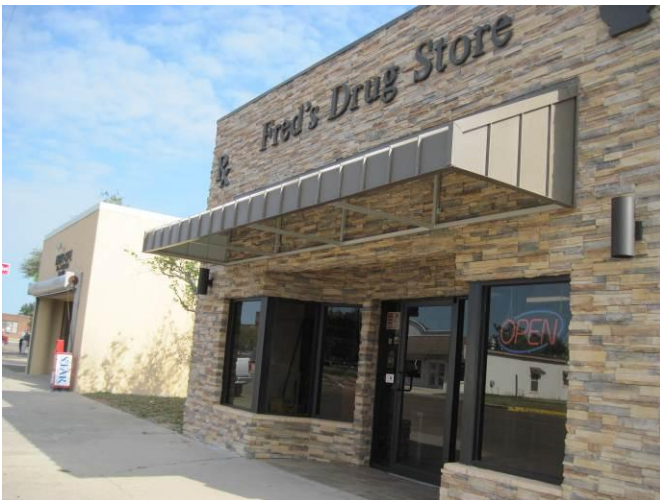
1935 pharmacy/soda shop renovated to Texas vernacular style.
