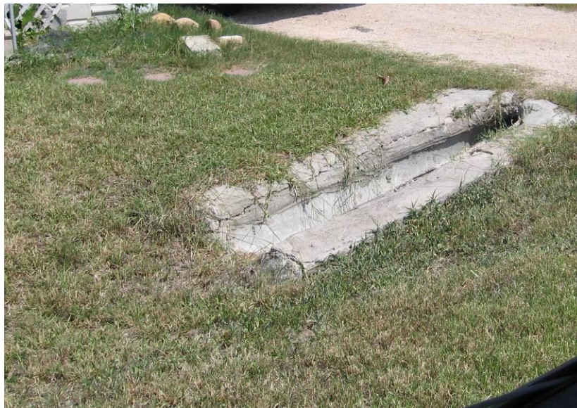
Figure 7F. Culvert with Safety End Treatment (SET) in good condition
