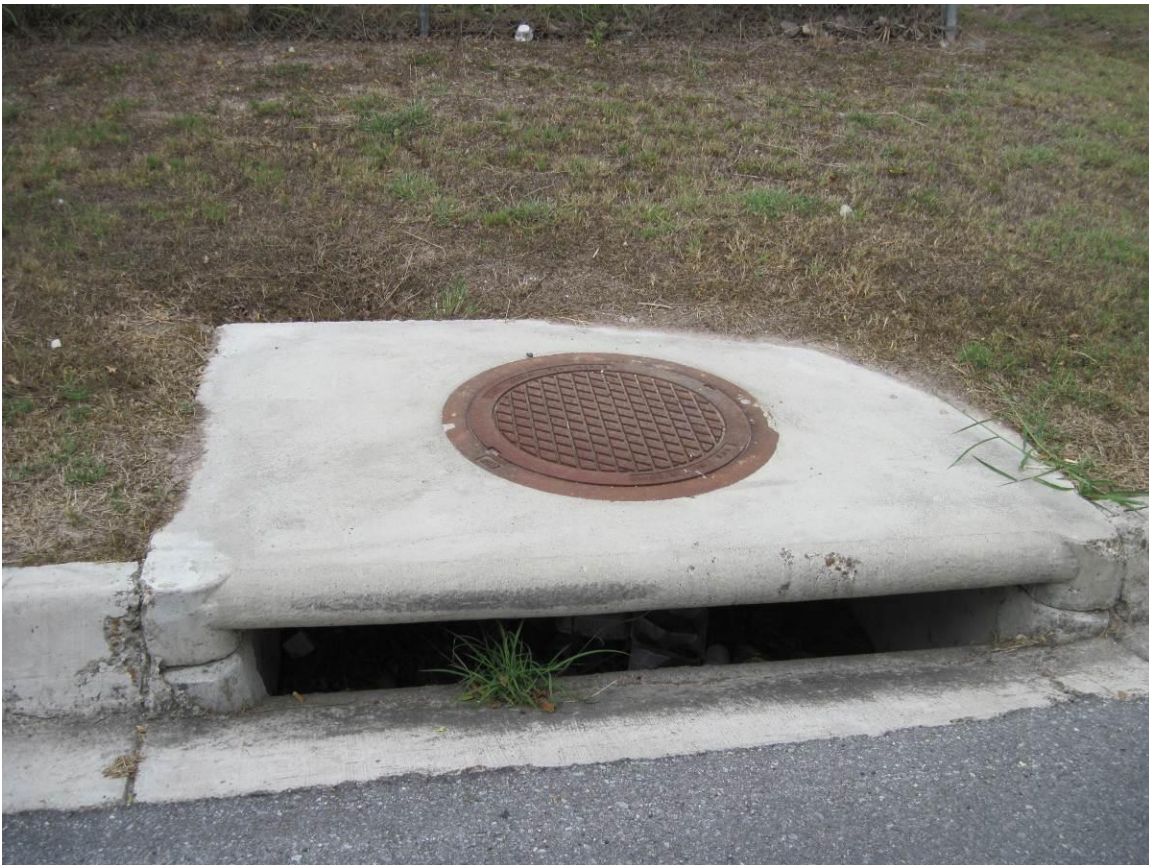
Figure 7C. Curb Inlet in good condition
