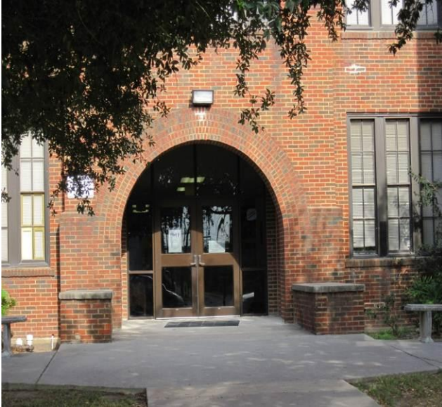
Original school building features 1900-style Victorian archway.
