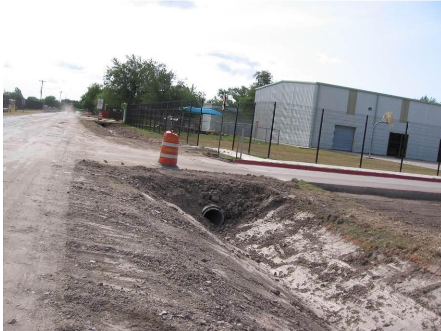
Figure 7E. Culvert w/o Headwall in fair condition
