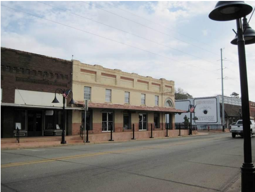
Wiring in Hughes Springs, Texas CBD doesn't interfere with building lines; decorative street lighting placed as part of a Downtown Revitalization Project provides illumination at night at the awning level
